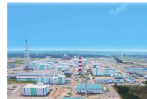
Rokkasho Reprocessing Plant
